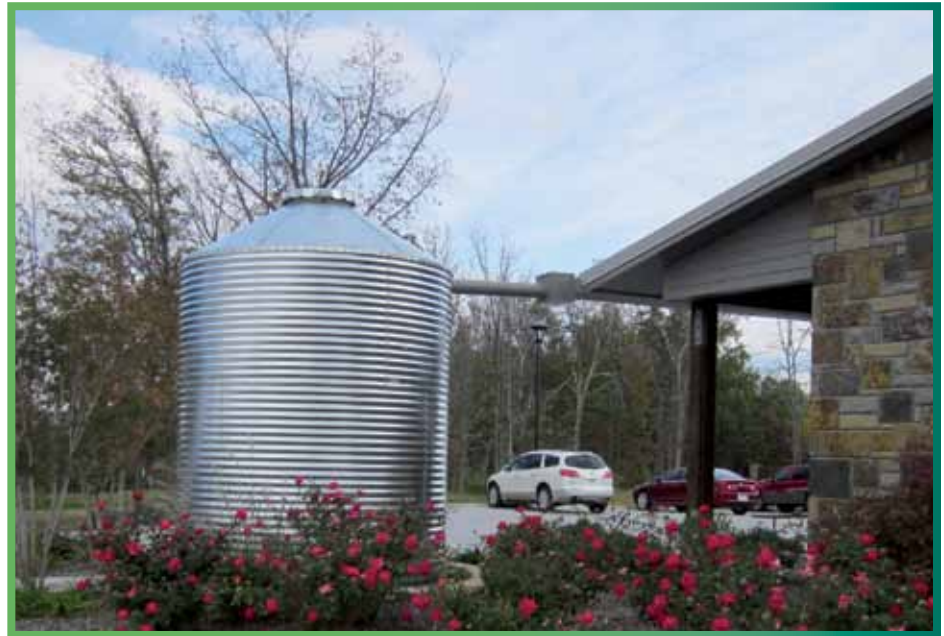
The exterior barn motif of the building complements the neighborhood of Riley Farms. A silo collects rain water that is used for flushing the toilets.
